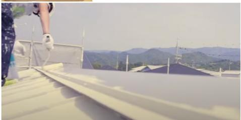
Regarding the painting method, do not only apply in a certain direction, but be sure to pass it vertically and horizontally. (The special aggregate will be biased and the finish will be poor.)
